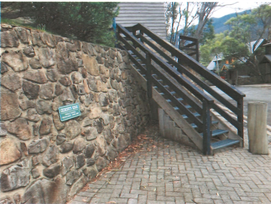
Photo 2 General street view of Flight 1 and retaining wall
