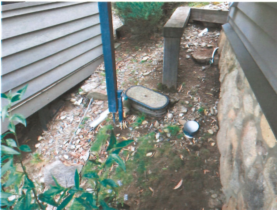
Photo 1 Between the two lodges, east side. Note comms (?) cover.
